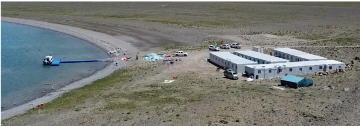
Fig. 6: Overview of the NamCore camp, including the pier (left) and containers equipped for living (right)
